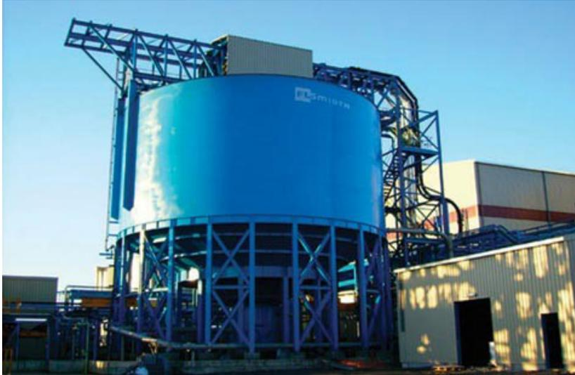
Figura 8 – Deep Cone Paste Thickeners/EIMCO
