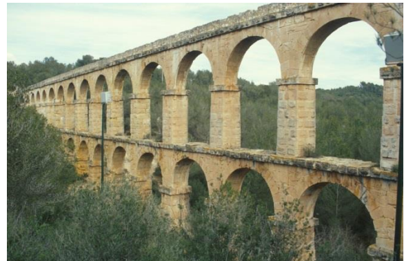
Figure 2. Aqueduct near Tarragona (Spain).
