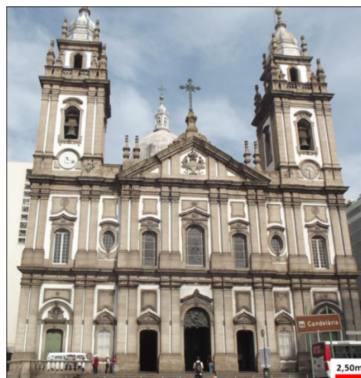
Figura 1B. Fachada Principal
